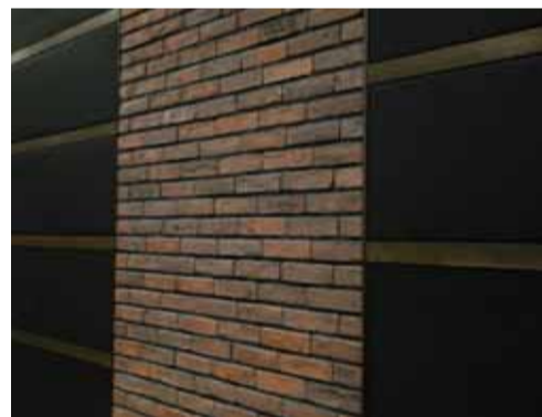
遮音と吸音の壁造作
