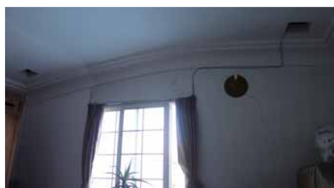
3階自宅の漆喰壁
